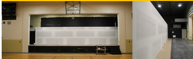
Hamilton Middle School East Gym Stage Improvements (2023 Bond)
